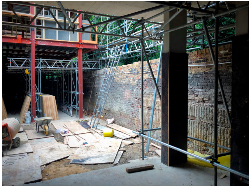
Courtyard space under construction
